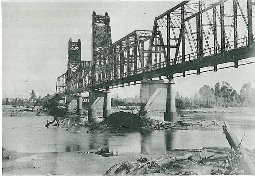
The Index Bridge as it looked in 1921. The picture was made to illustrate the problem of drift around the piers.
